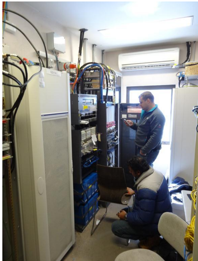
Figure 12: Existing communications room fit out, to accommodate Vodafone upgrade.
