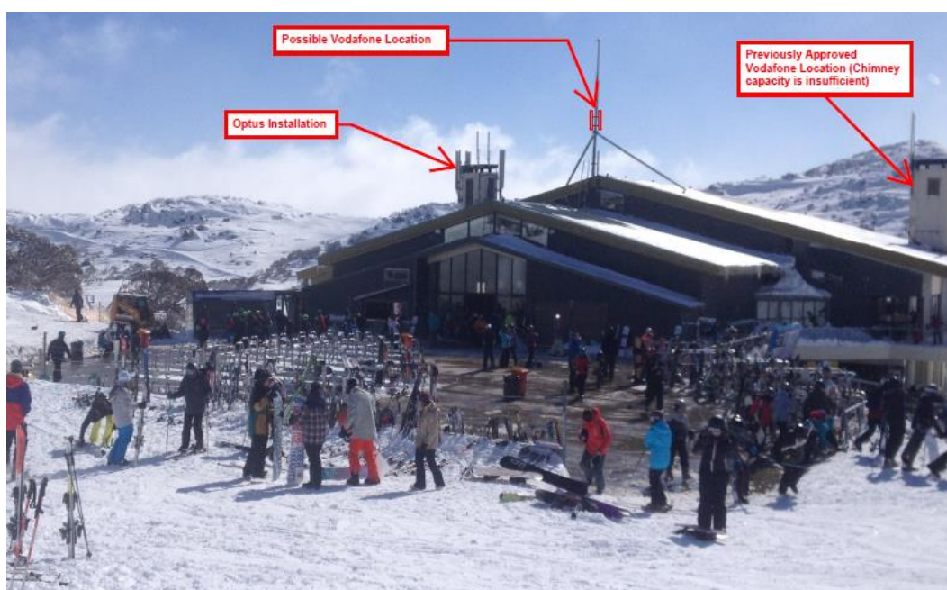
Figure 2: Blue Cow Ski Terminal Building
