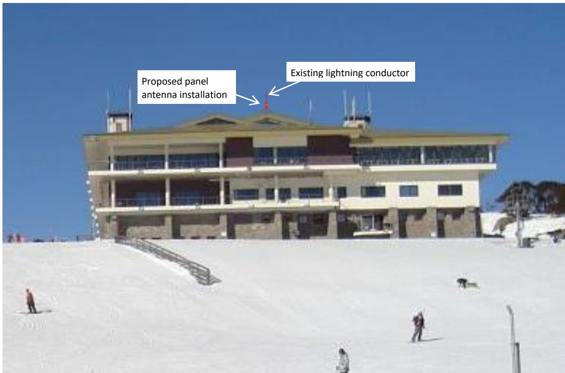
Figure 9: Expected visual impact, as per the northern building aspect. Antenna installation impacts are minimal from 65m. Installation will be colour matched 'gull grey'.
